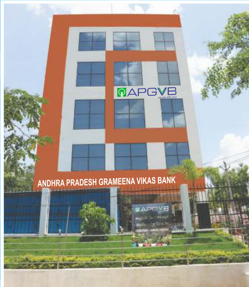
Newly constructed own spacious Building for Staff Learning Centre with residential Accommodation, Regional Office & IT Cell at Sangareddy
